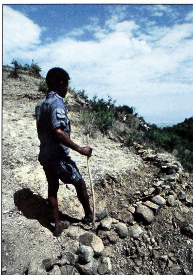
On weekly community work days, everyone turns out to help build simple hillside terraces for capturing topsoil and rainwater runoff. Villagers will plant trees along each contour when the rainy season begins.
